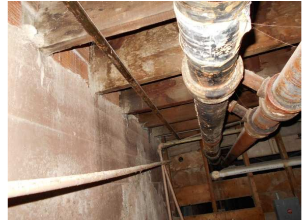
Photo 11: First floor joists embedded in exterior clay tile walls supported on concrete basement walls.
