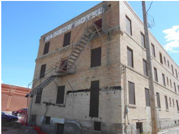
Photo 19: North and west walls. Brick veneer in good condition.
