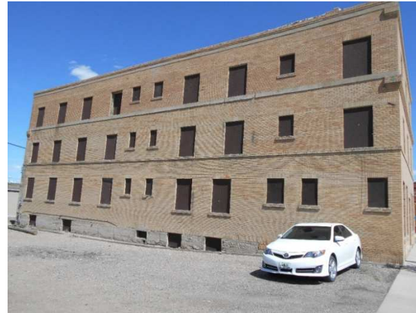
Photo 21: West wall. Note at-grade basement windows and flat site grading.
