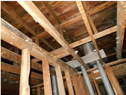
Photo 8: 2x6 roof joists are supported by 2x cripple walls which are carried by 2x10 ceiling joists.
