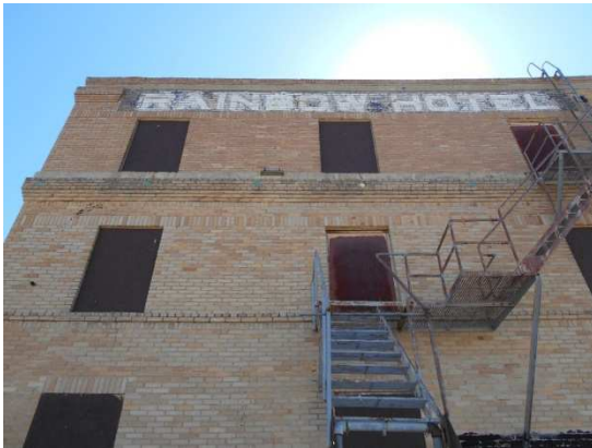
Photo 2: North wall of Hotel Building.
