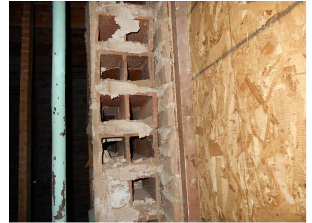
Photo 17: Exterior clay tile wall with brick veneer.
