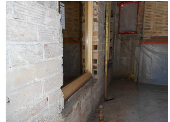
Photo 17: Exterior clay tile wall with brick veneer.
