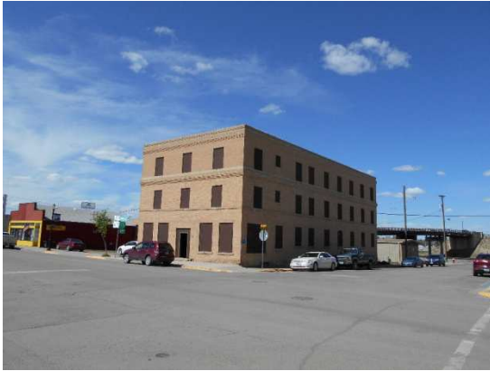
Photo 1: Exterior view of front (south and east) walls of the Rainbow Hotel.
