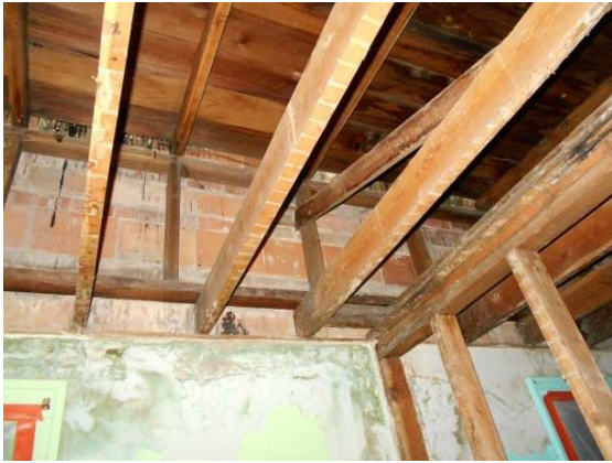
Photo 7: Ceiling and roof joists at exterior wall.
