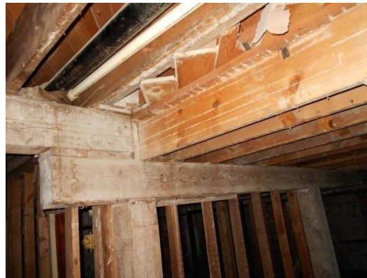
Photo 10: 2x12 floor joists supported on timber beams and columns in the basement. Floor elevation steps above.
