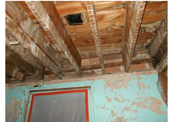
Photo 6: Third floor ceiling and floor joists supported on exterior clay tile wall.
