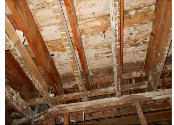
Photo 5: Third floor ceiling joists (below) supported on corridor bearing wall. The flat 2x member transfers load from the floor joists (above) to the ceiling joists.
