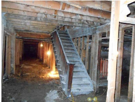
Photo 9: Looking south down center corridor in basement. Rows of beams and columns on either side support interior bearing walls above.
