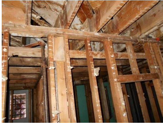
Photo 3: Second floor joists supported on interior corridor bearing wall.
