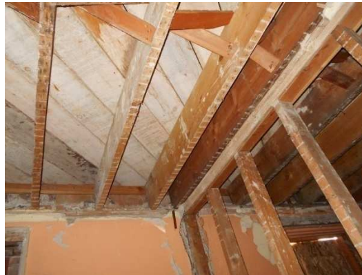
Photo 4: Second floor joists supported at exterior clay tile wall.
